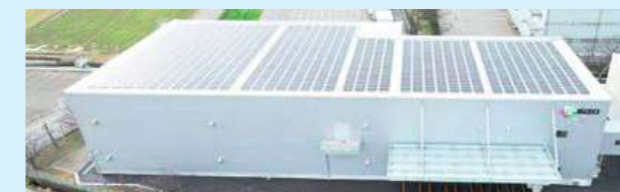
EIZO Corporation Logistics Building (FY2022)
